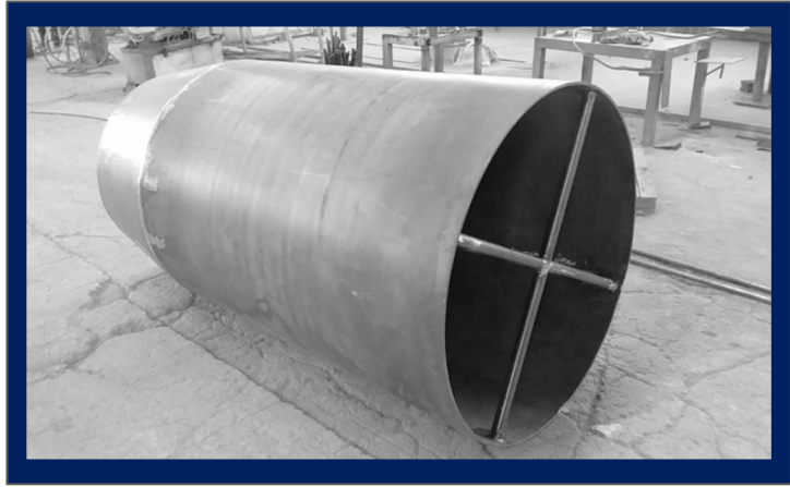
Manufacture of falsework, shovels and chisels.
