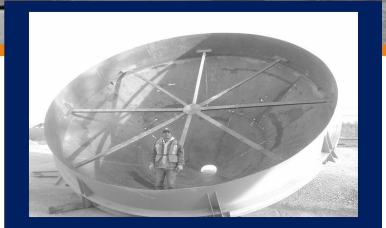
Manufacture and assembly of silos.
